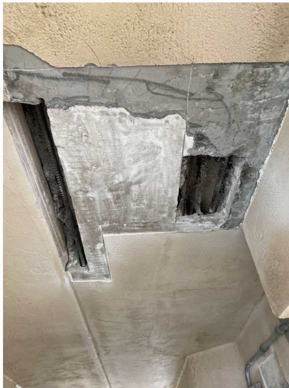
Picture 6: Typical ceiling excavations on the walkways
