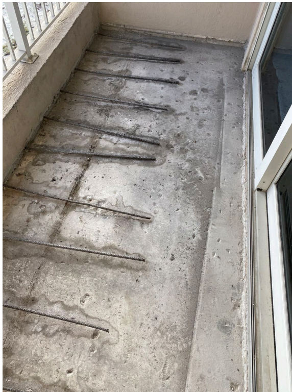
Picture 2: Typical topping replacement
