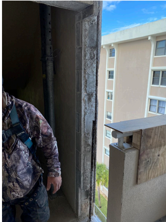
Picture 3: Typical wall repair on walkways
