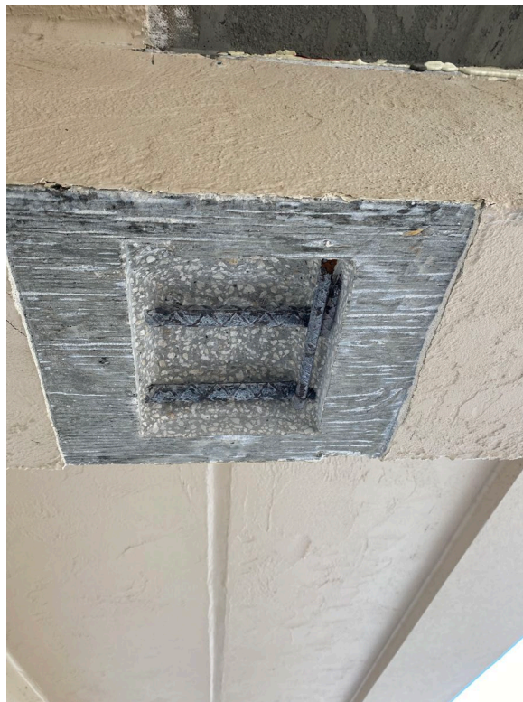
Picture 4: Beam excavation on the walkways
