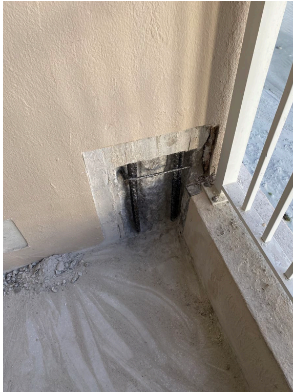
Picture 1: Typical wall repair
